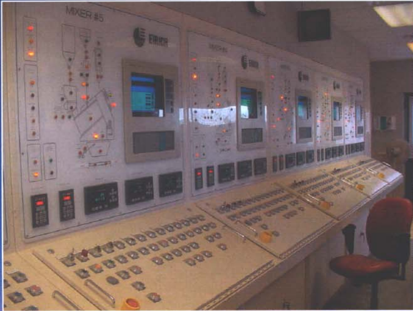
Figure 1. Custom interface electronics, networked controller and automated on-screen indicators.
