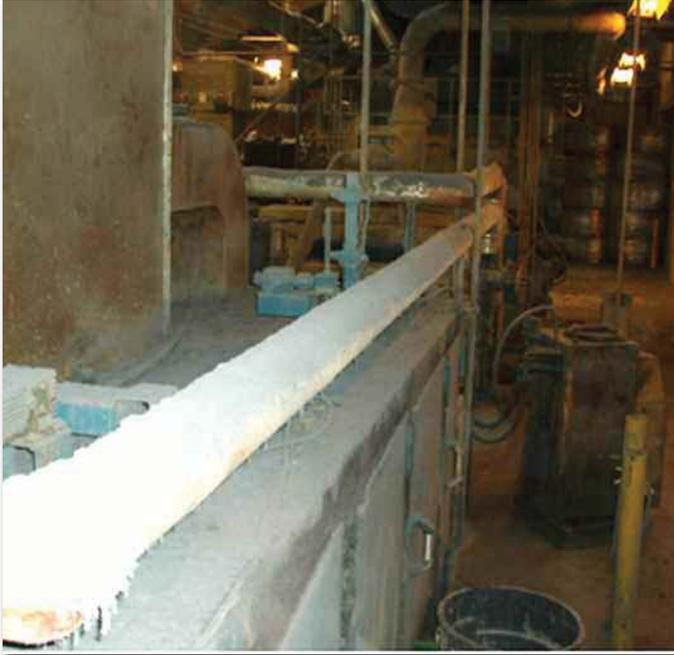
**Photo 3: Phenolic resin dust accumulation due to inadequate dust collection.**
