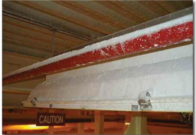
Photo 1: Dust accumulating on overhead surfaces.
